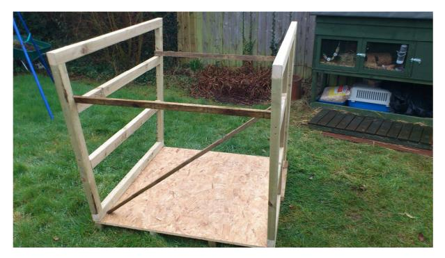
**Step 5** - Measure between ends and make side frames. Make both sides the same with sloping middle timbers. This will be where the slanted windows with fit. The same technique can be used where you lay the middle timbers on the outer ones and mark off the angle wanted.
