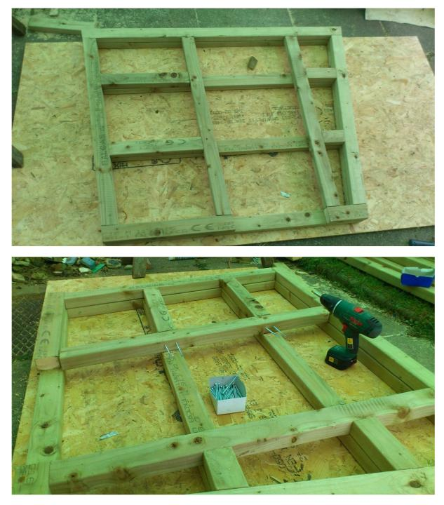
**Step 4** - After screwing together the frame place on plinth and fix down using 100mm 10s screws. Use pieces of batten to brace and hold in place.
