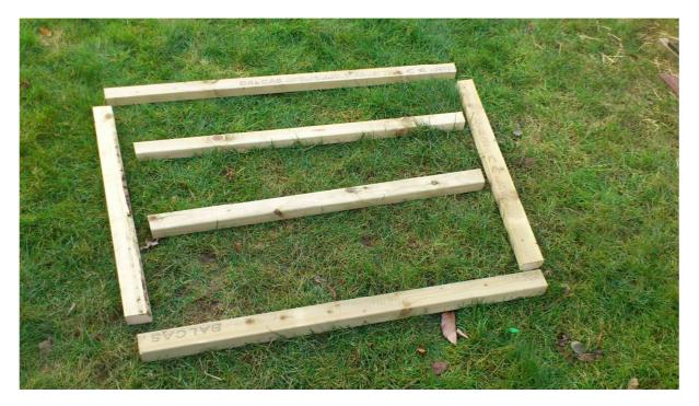
**Step 3** - For the front frame lay the timbers on the rear frame so you get the same size. Mark out the size of door with a straight edge and cut timbers. Again fix together with 100mm screws.
